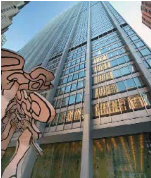
Milbank's 330,000-square-foot headquarters at One Chase Plaza in Lower Manhattan.
